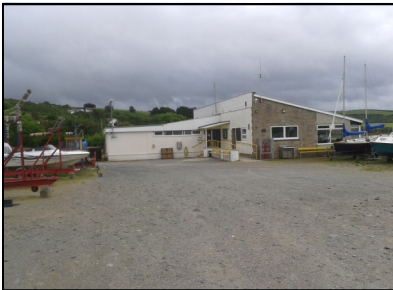
The Teifi Boating Club before, during and after extension work
