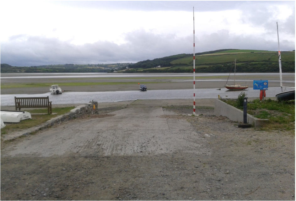
Teifi Boating Club slipway and estuary at low water
